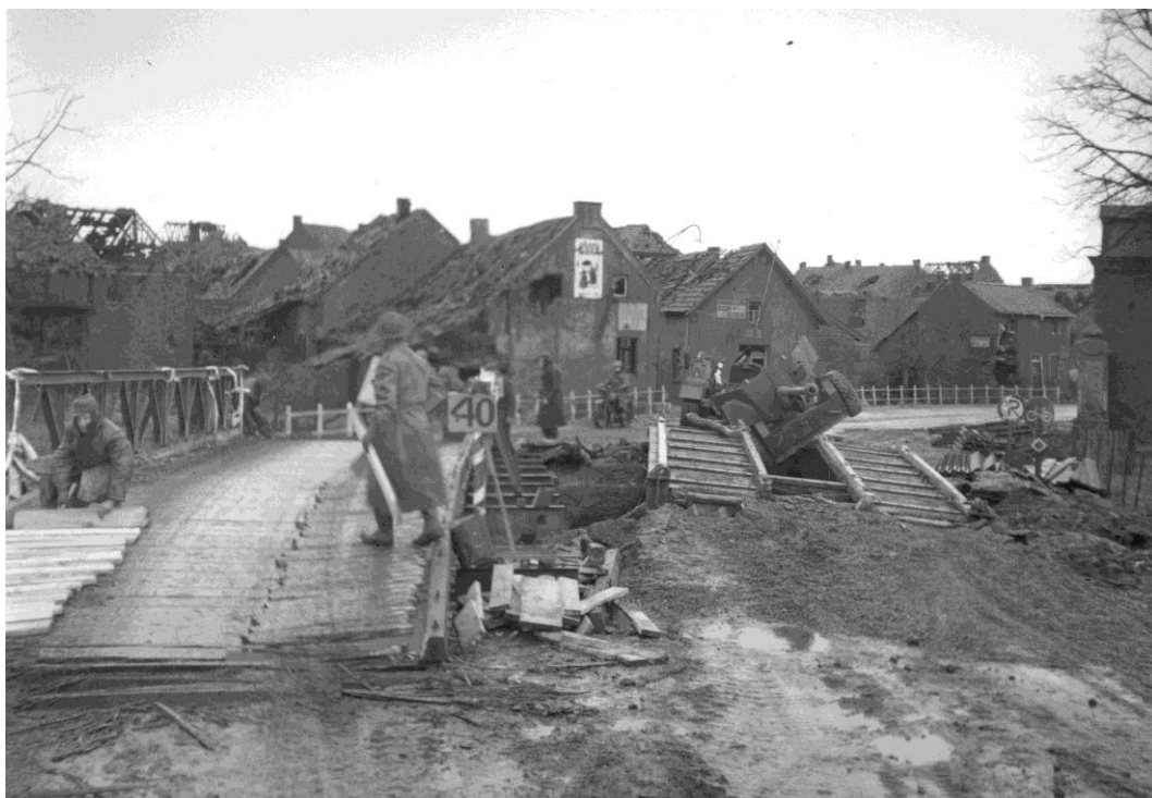
621 st Royal Engineers Laying Chessing On Bailey Bridge At Susteren, January 1945
